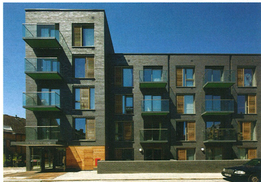
Darling Associates' Fermoy Road housing in London for Pocket Living comprises 32 one-bedroom units.
